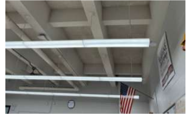
Typical Concrete Framing in Classrooms
